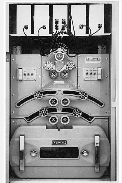
Elliott 405 magnetic disc (16K words)
