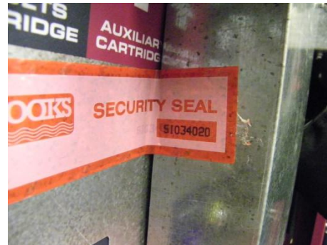
Figure 22: Sticky adhesive tape seal
