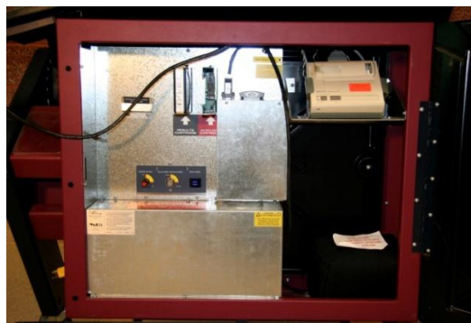
Figure 2: Rear of AVC Advantage cabinet with door open (hinge at right)
