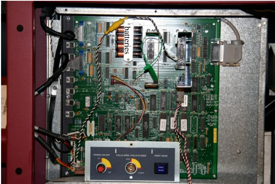
Figure 4: Circuit-board cover removed from motherboard enclosure. Bottom center, panel for on/off knob. Top center (just to the right of "batteries"), a green strap seal remaining after the circuit-board cover has been moved past it (see discussion of "seal regime #1"). Slightly to the lower right of center, 1 configuration ROM and 3 program ROMs with white labels. At top left and top center of enclosure, one can see two of the 10 threaded holes for the screws that hold the circuit-board cover in place.
