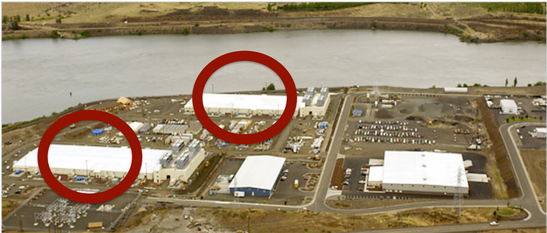
Google's datacenter in the Dalles, Oregon (350k servers) Each the size of a football field!
