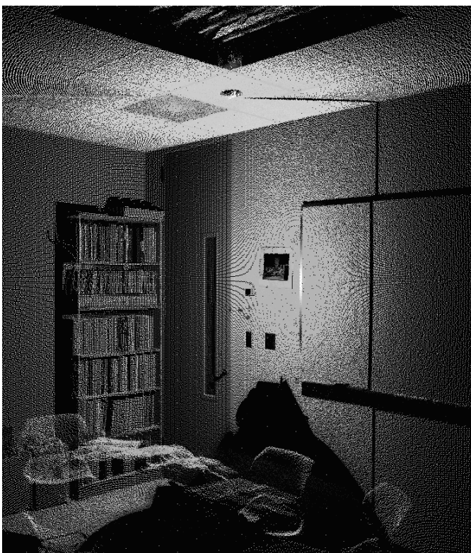
Fig. 11. View showing a break in the ceiling where the counter-clockwise scans meet the clockwise scans, showing the seam where data is missing due to errors in the panning unit.
